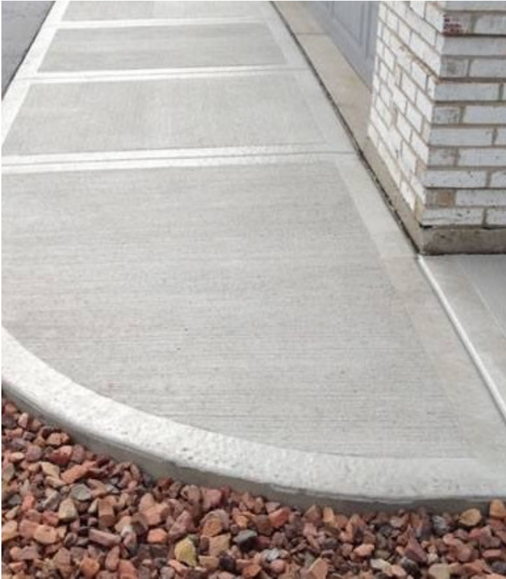
insitu concrete surfacing brushed finish with smooth edges - main public footpath material
